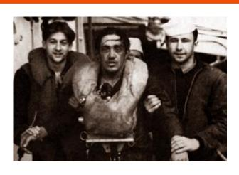
During World War II, submariners on German U-boats were able to leave disabled vessels if the boats were sinking in relatively shallow water. To help them breathe, U-boat crew members wore a Dräger Lung (similar to a Momsen Lung which was used on U.S. boats). This U.S. Coast Guard picture shows a German U-boat survivor who had escaped from U-175. He is wearing a Dräger Lung.
