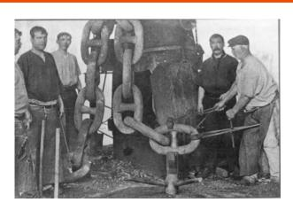
Ten teams of chain makers worked on *Titanic's* anchor chains. Those chains were 3 3/8 inches in diameter. Note the cross piece on each chain link. It is called a "stud link chain." That middle bar is intended to stop the link from kinking or from deforming if it is under a heavy load. This 1911 photograph appears in <u>Chain and Anchor Making in the Black Country</u>, a 2006 book by Ron Moss.
