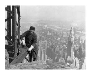
As a photographer for the Federal Works Agency, in 1930, Lewis Wickes Hine took this photo of a worker fastening bolts on a beam of the Empire State Building during its construction. The photo is <u>online via the U.S.</u> National Archives. Click on it for a full-page view.
