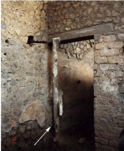
Boscotrecase. Repairs of damages caused by pre-eruption earthquakes.
