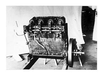
The Wright Brothers used a 12-horsepower engine for their first powered flight. This image depicts the actual engine. NASA tells us it had the equivalent power of "two hand-propelled lawn mower engines." Image online, courtesy NASA.
