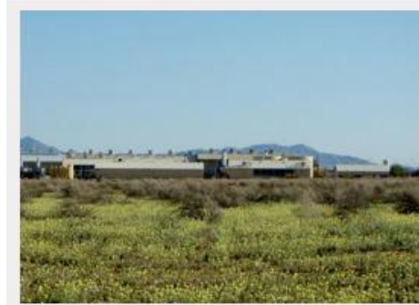
PG&E's Hinkley natural gas compressor station near Barstow, California
